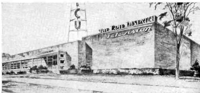
WICU (TV) building now under construction.
